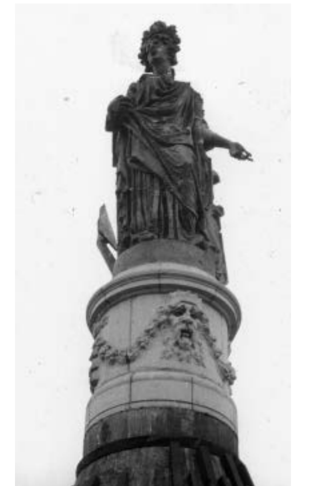
Custom House, statue of Commerce on nearly completed new dome, 1928 IAA T.J. Byrne Collection 2012/51.1/51
