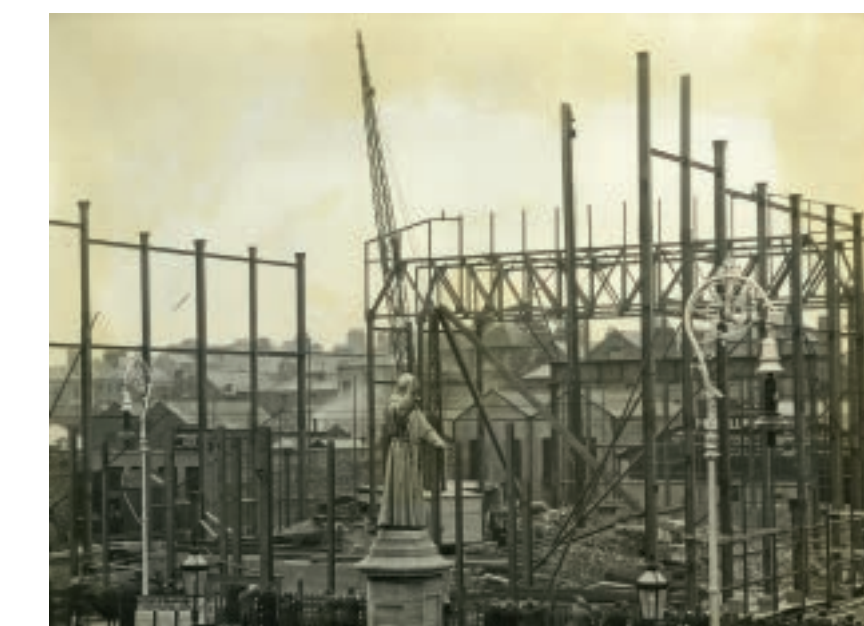
Savoy Cinema, steel frame under construction, September 1928
