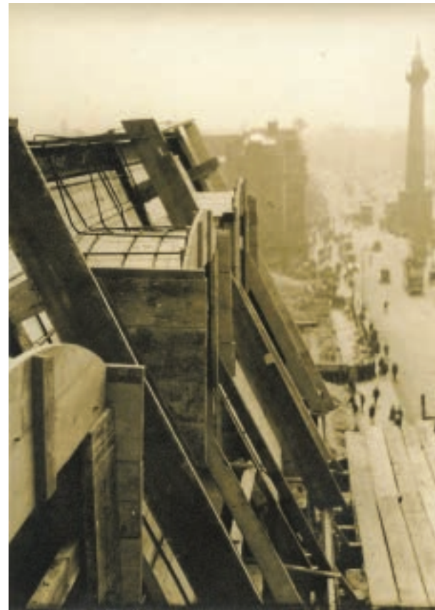
O'Connell Street, Upper, Gresham Hotel under construction, 1927
