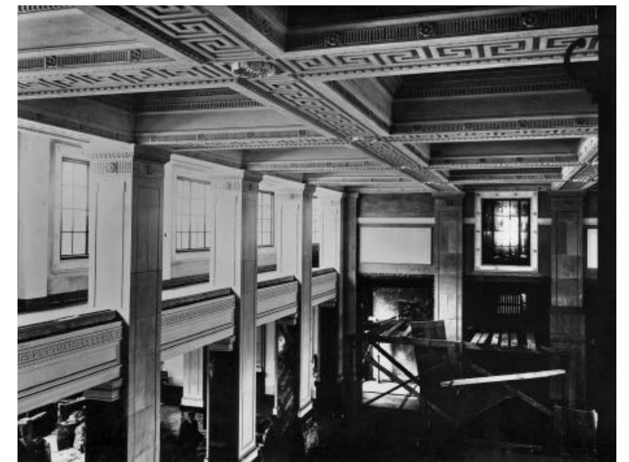
View of public office of new GPO nearing completion, 1926 IAA T.J. Byrne Collection, 2012/51.6/3
